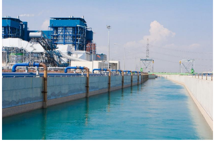
Figure 1 - Wastewater treatment at a petrochemical site
